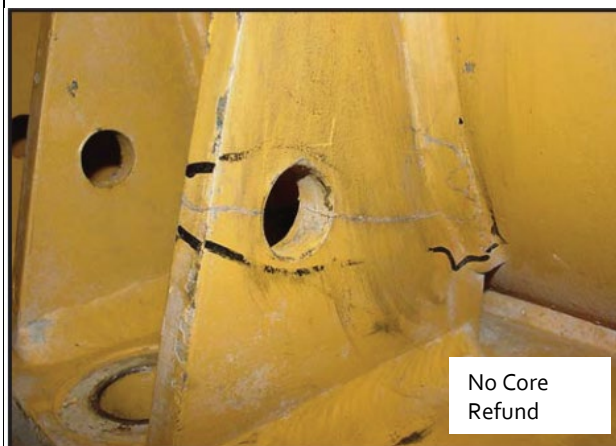
Figure 9 - Visibly cracked or broken
