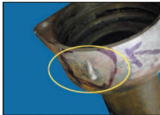
Figure 7: Non-operational damage - melted by torch
