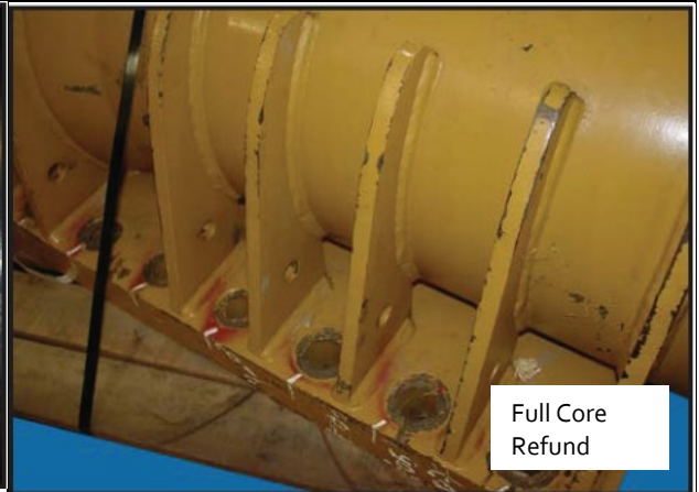
Figure 8 - Not visibly cracked or broken
