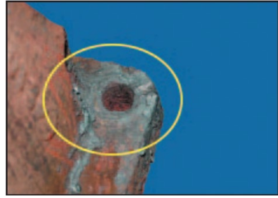
Figure 6: Non-operational damage - melted by torch
