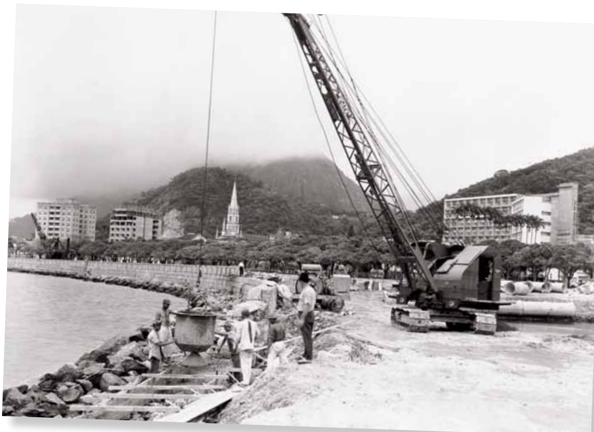
Cat and Bucyrus products have made immeasurable contributions to the mining industry—and the world. Above, a Caterpillar D4600 engine powers a Bucyrus Erie crane, which is being used to build a sea wall in Rio de Janeiro, Brazil, in 1949.
